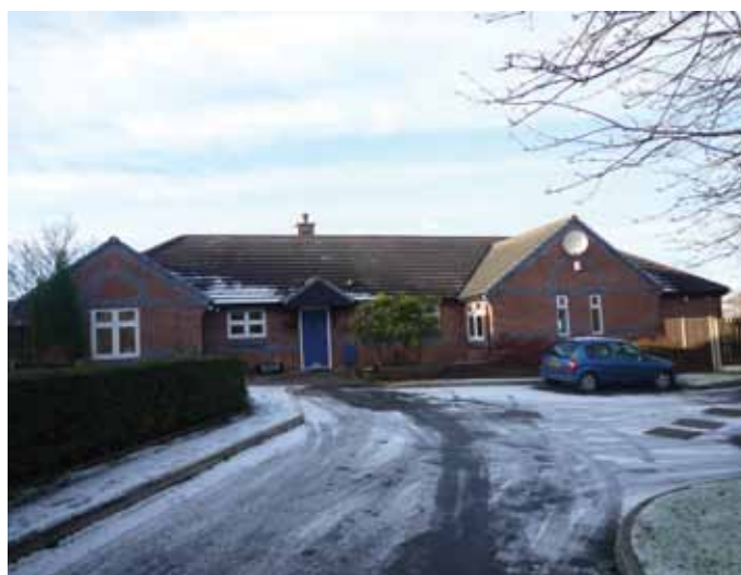
Malton Drive is a residential care home meeting the needs of six adults with learning disabilities
